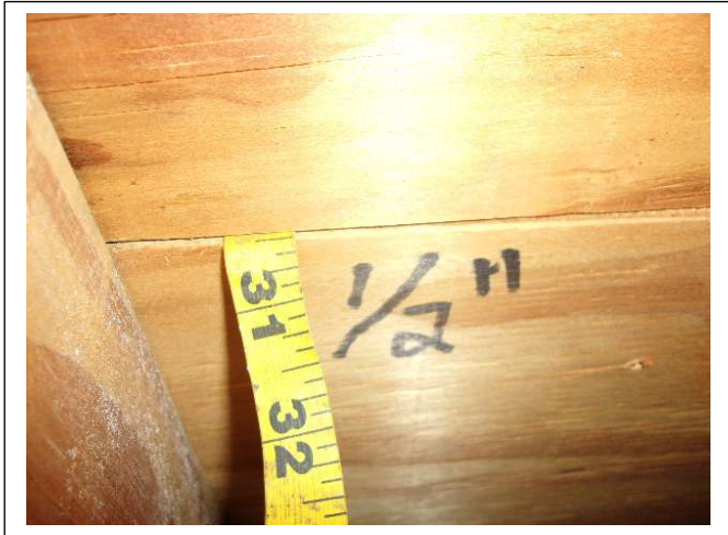
ROOF DECK THICKNESS – ½ inch plywood
