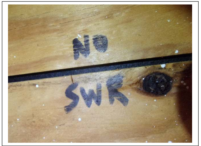
SECONDARY WATER RESISTANCE – Is not installed
