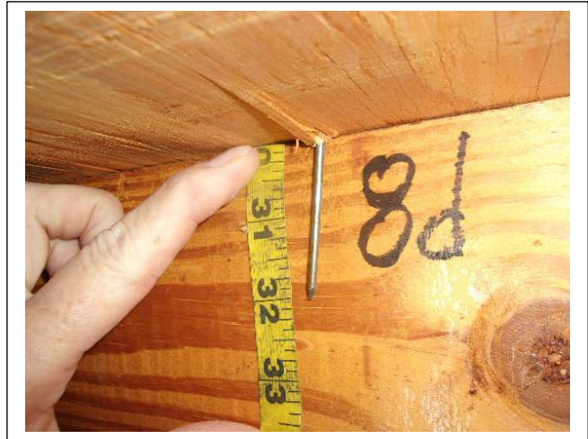
ROOF DECK ATTACHMENT – 8d nail
